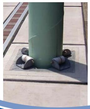
Galvanized steel pile ring is embedded into the concrete surface. Ultra high molecular weight plastic rollers on stainless steel pins are used to ensure smooth maintenance free operation.
